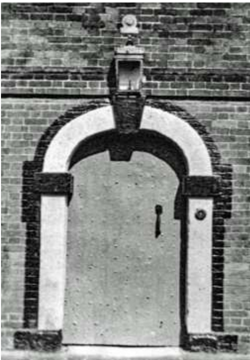
Front door of Wimborne Workhouse Courtesy of the Priest's House Museum Collections Trust
